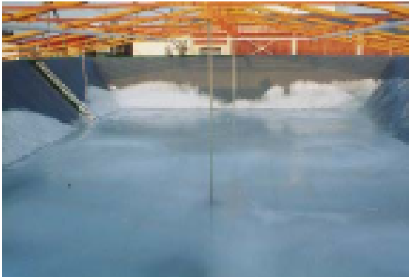
Photo 1: The ice pond in operation.
